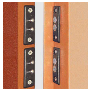
Double electrical contacts between leaf and doorframe
